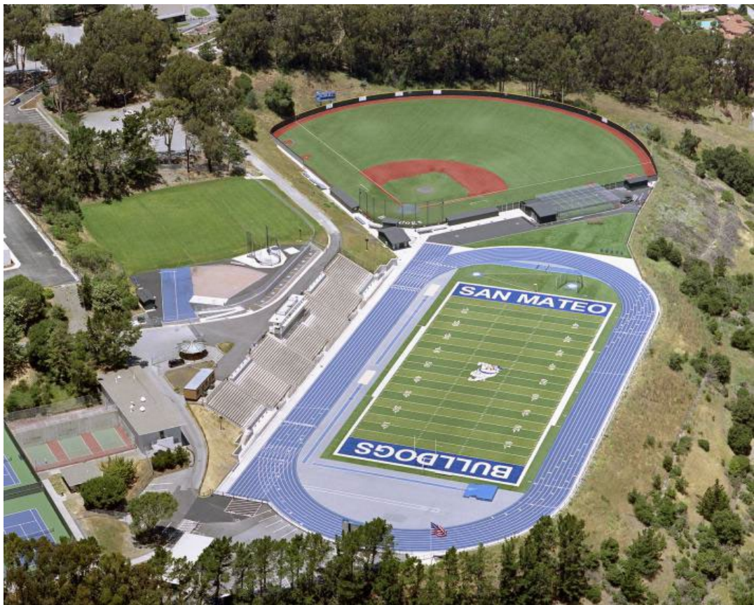
22 Completed San Mateo Athletic Facilities
